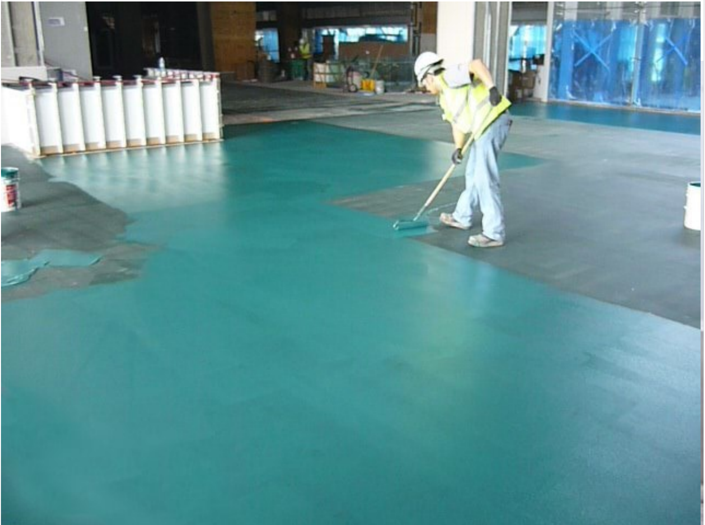
MAPEI Project: Dallas Cowboys Stadium, Arlington, TX
