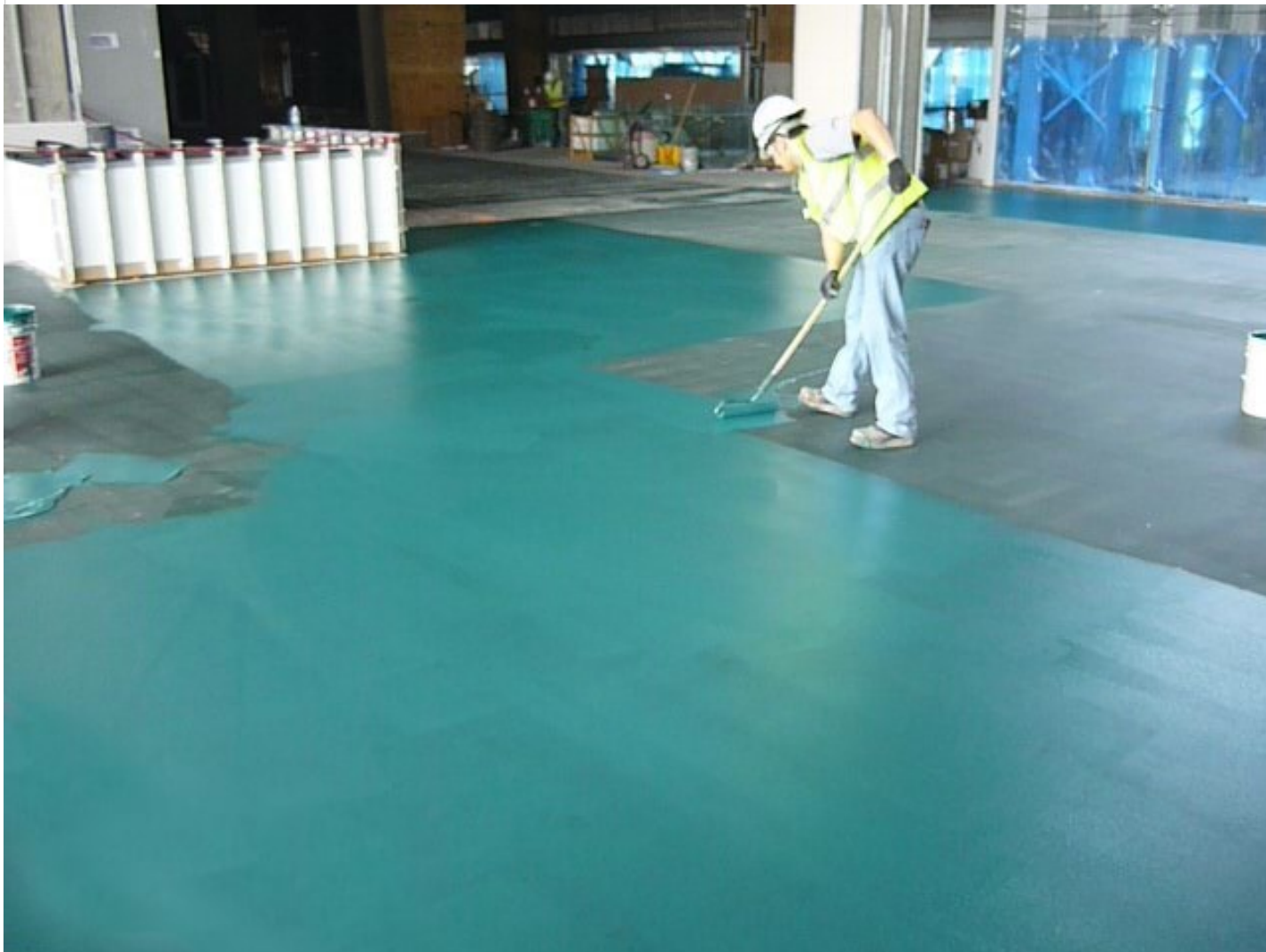
MAPEI Project: Dallas Cowboys Stadium, Arlington, TX
